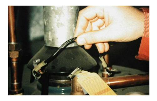
Flue gas spill switches normally connect to the gas valve on gas fired appliances and the switch will shut the valve after sensing flue gas spillage such as that which could occur if the flue becomes blocked.
