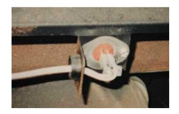
Older heaters with no flue spill switch: On older heating systems these safety switches may not be installed at all. A spill switch or a set of them
