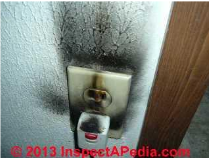
Our photo (above left) illustrates a burned-up electrical receptacle whose circuit was protected by a Zinsco circuit breaker that failed to trip and in fact had burned itself in the panel.
